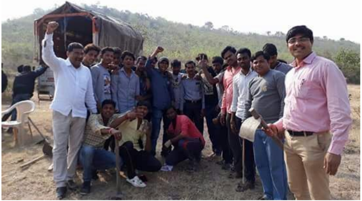
Happy faces after constructing Contour Trenching for Water Harvesting on Hills during camp.
