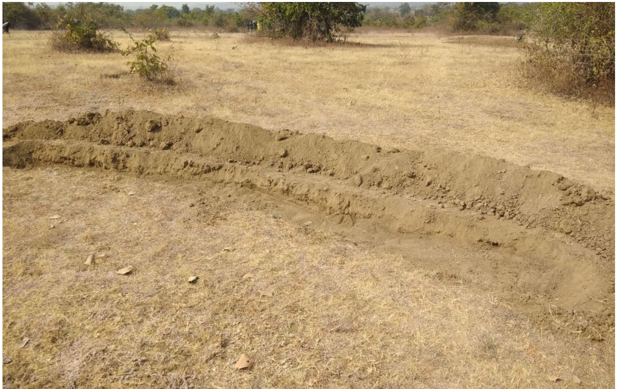
Contour Trenching for Water Harvesting on Hills during camp.
