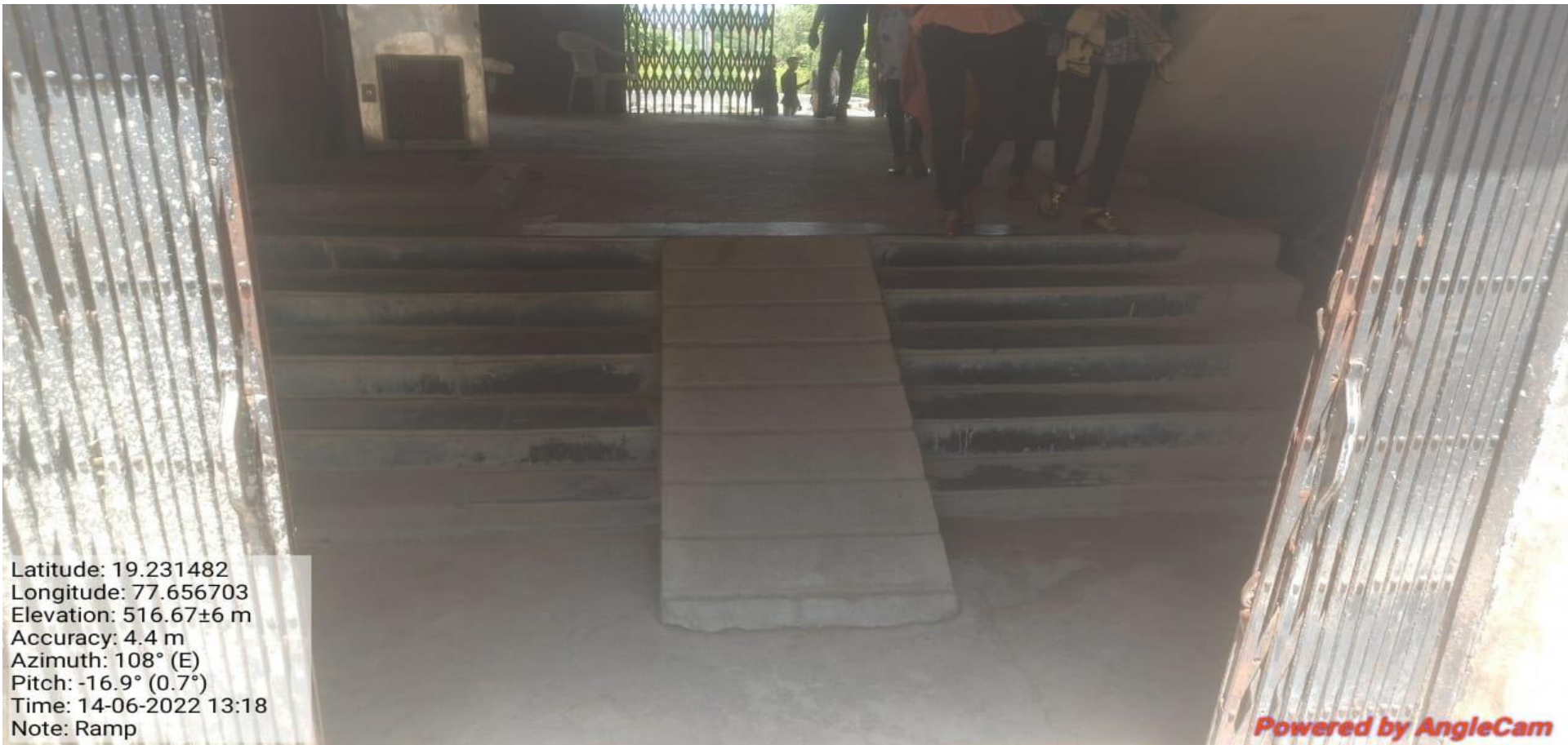
Ramps at the Back Entrance
