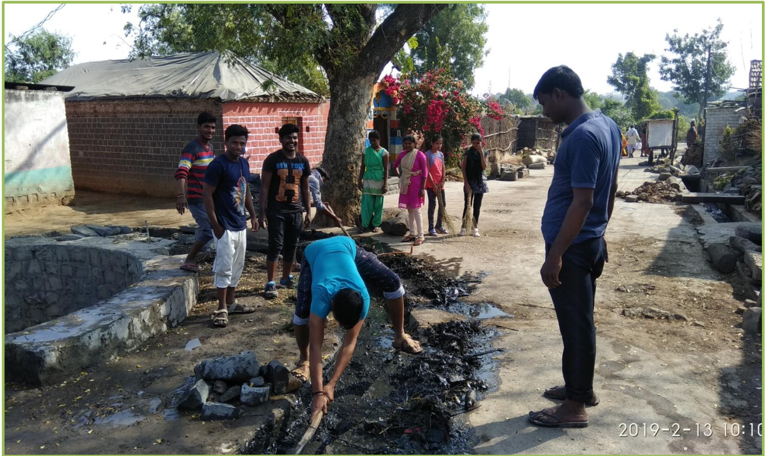
Drainage water management by nss volunteers
