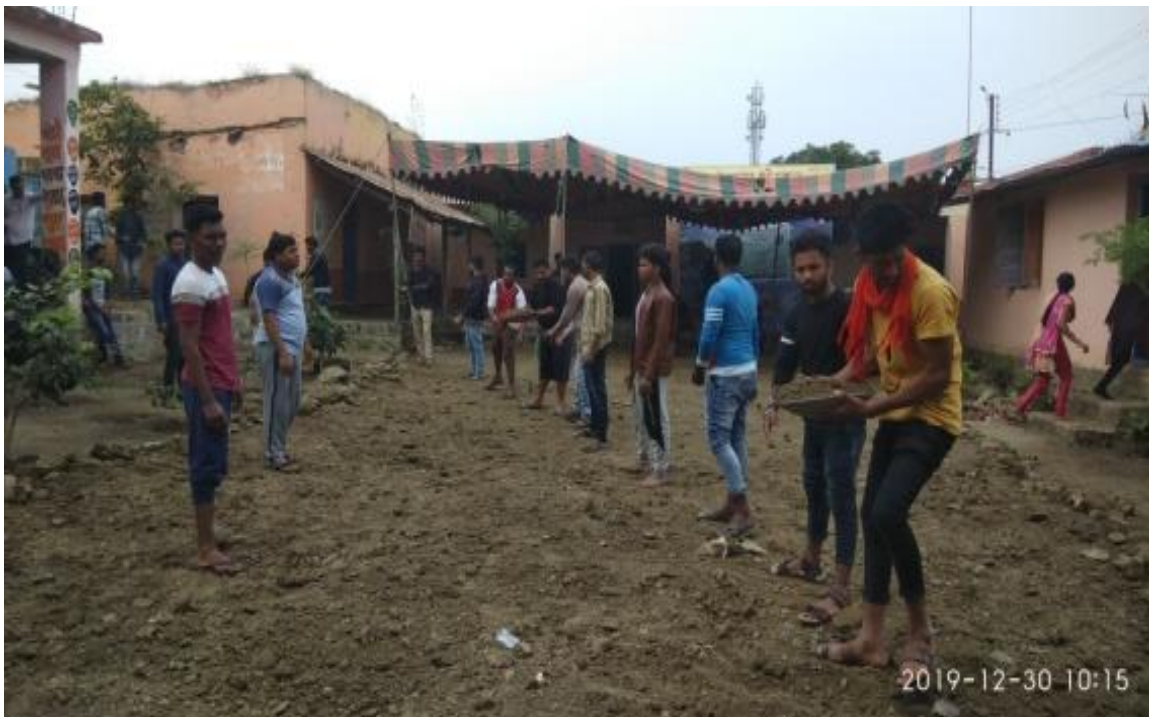
@ ZP School – Preparation of Playing ground for children.
